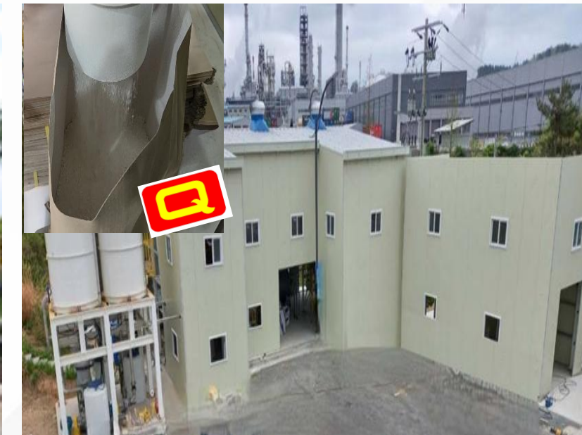
Indirect carbonation PP (2TPD)
