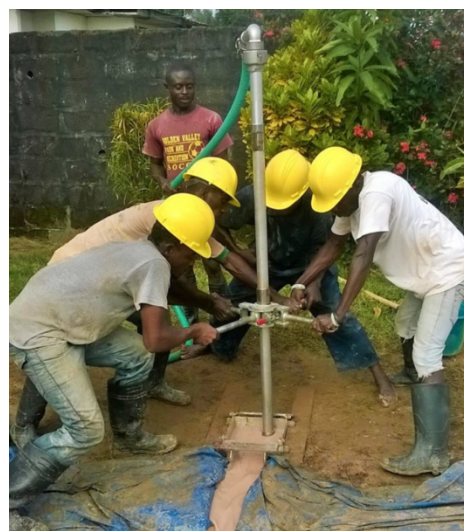
Figure 2. Manual drilling team using the jetting technique.
