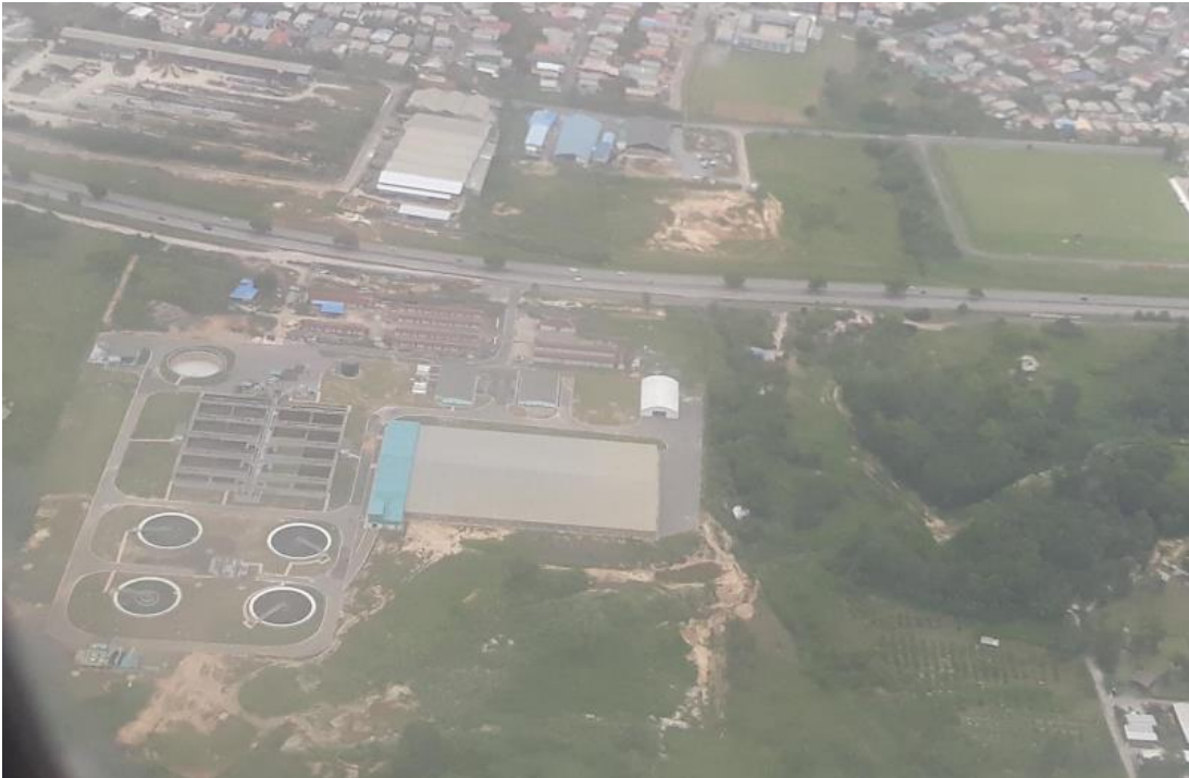
Plate 3 WASA Malabar Wastewater Treatment Plant
