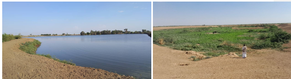
Figure 13. Left: The recharge basin during the wet season, showing full storage of diverted floodwater (Source: Plan International). Right: The same basin during the dry season, where vegetation growth indicates moisture retention and localized groundwater recharge (Source: field work 2024).
