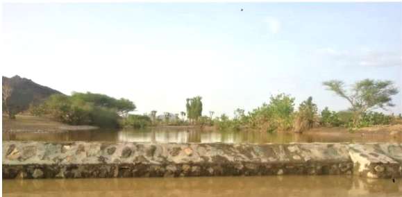
Figure 1, The Anikwan sand dam in Red Sea State shortly after the rainy season. The masonry structure spans the wadi channel, retaining runoff and coarse sediment to enhance infiltration and sustain groundwater recharge in the dry months.
