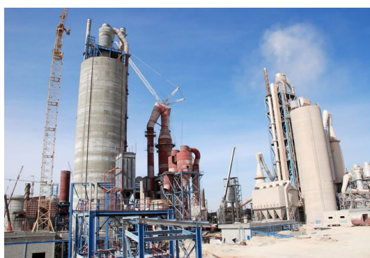
Figure 18 Atbara Cement Factory, River Nile State
