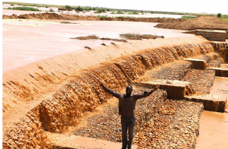
Figure 13 Water Spreading Structure in North Darfur. Source: UNEP and Practical Action
