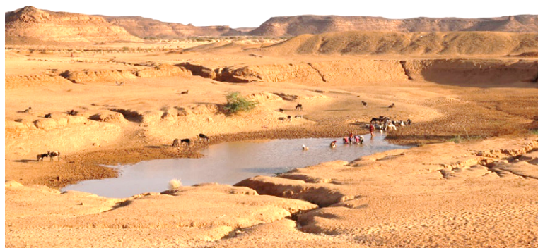
Figure 5, the Great Hafir, Muswarat, River Nile State. Dates 2500 years ago harvesting water from Wadi es-Sufra and has a capacity of 260,000 m 3 .
