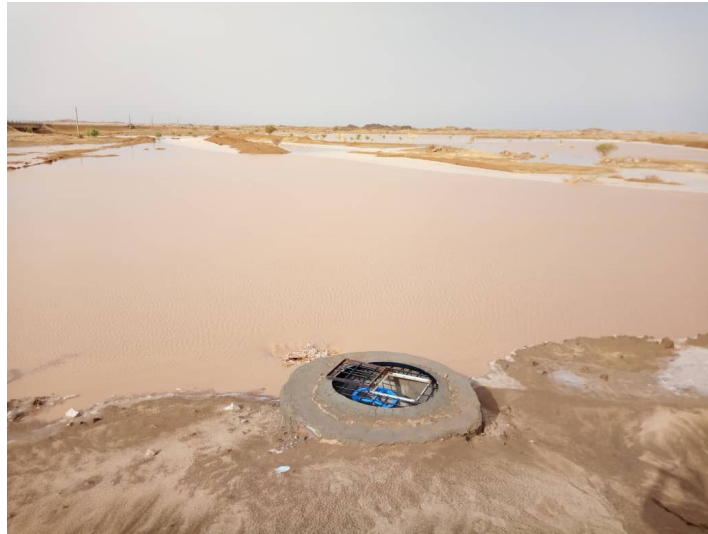
Figure 25, Improved road water harvesting, Haya, Red Sea
