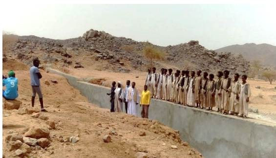
Figure 20 Reinforced concrete sand dam. Red Sea State. Source: SOS Sahel Sudan
