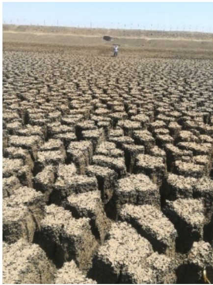
Figure 9 Excessive sedimentation in A Hafir in Al-Gadarif. Source: Consultant
