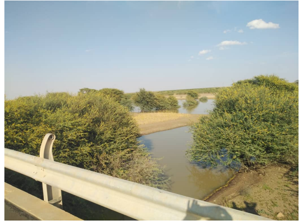
Figure 26 Upstream view of Alkassara road water harvesting. Source Field work 2024
