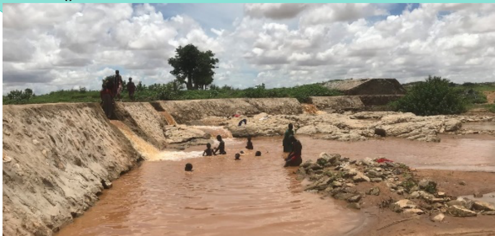
Figure 22 Baba sand dam, Nyala South Darfur. Source: ZOA International
