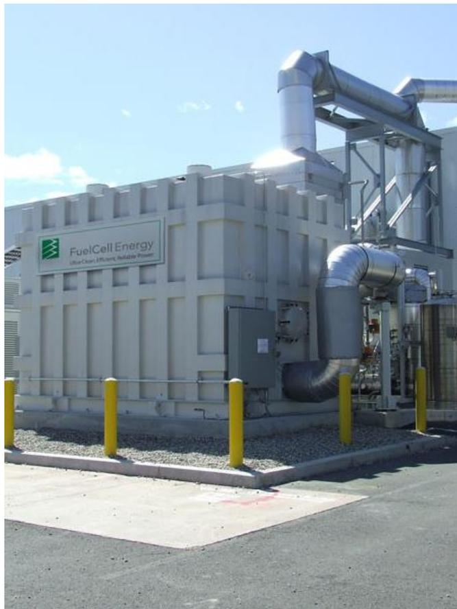
**Brief description:** Stationary fuel cell plants in industrial use cases typically generate power or combined heat and power (CHP) at MW-scale by converting natural gas, biogas or compressed hydrogen (from a grid or locally available), e.g. for electricity- (and heat-)intensive industrial production processes
