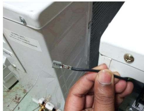
After: Connected in thimble, insulating sleeve
