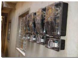
Conventional Meters enclosed in plastic to deter tampering
