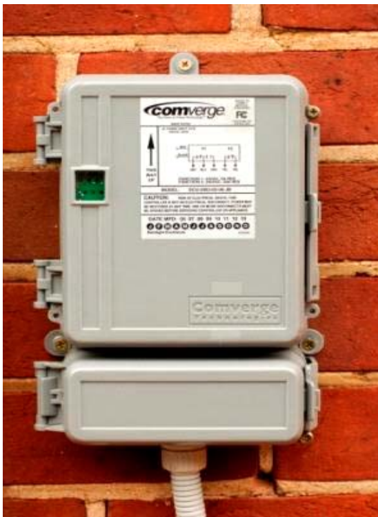
Figure DC06/2. Comverge Load Control Unit Used in the ETSA Utilities Air Conditioner DLC Trial
