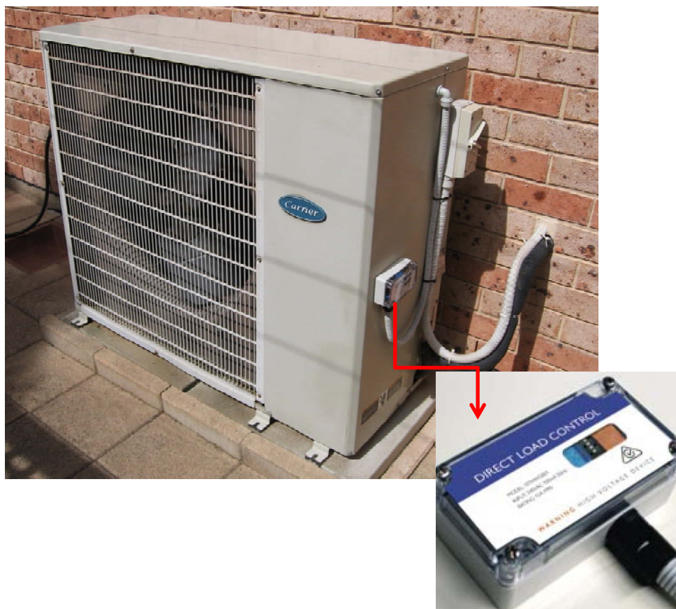
Figure DC06/3. Saab Systems “Peak Breaker” Direct Load Control Device Used in the ETSA Utilities Air Conditioner DLC Pilot Program
