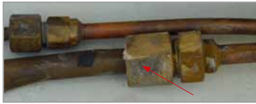
Figure 15: Mechanical connections in occupied space
