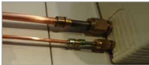
Figure 17: Joining tubes with Lokring couplers
