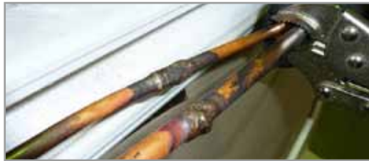
Figure 16: Removal of mechanical connections by joining tubes with brazing
