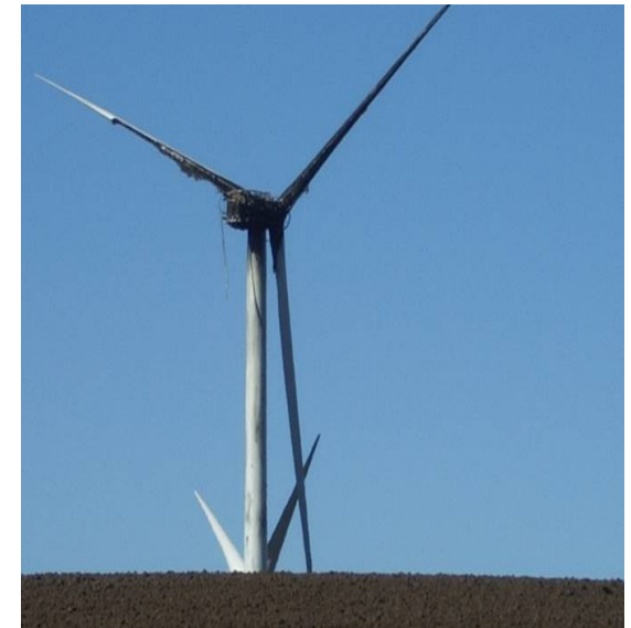
Wind turbine electrical fire at High Winds Wind Farm, Solano, CA (2004)
