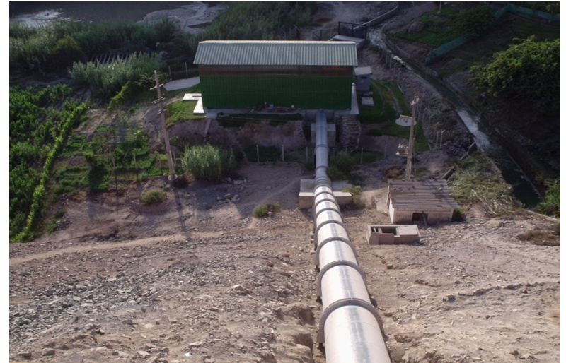
Santa Rosa Run-of-River Hydro, Peru, 5 MW
