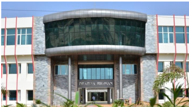
Figure 3: Front View of Prabha Bhawan (previously known as Design Centre)
