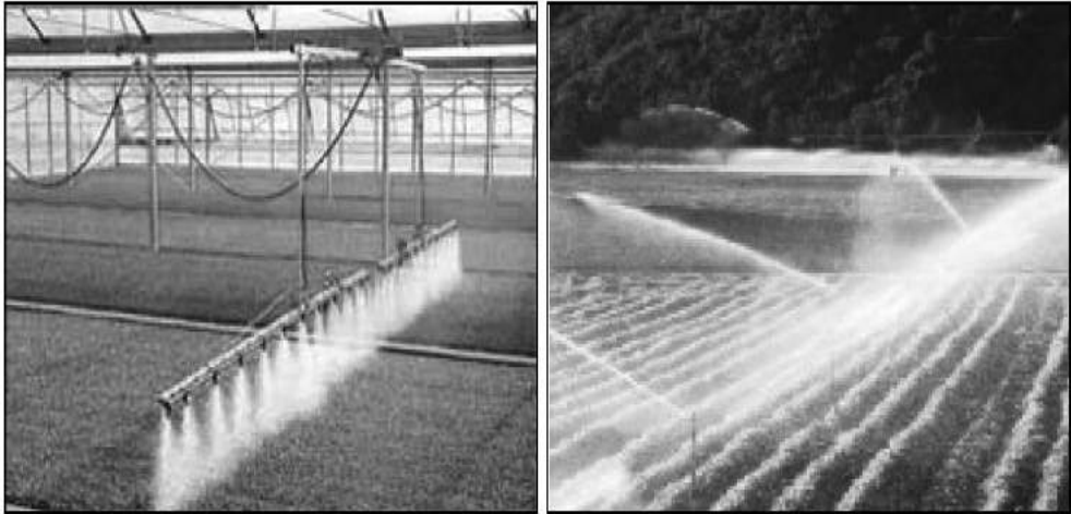
Micro irrigation system
