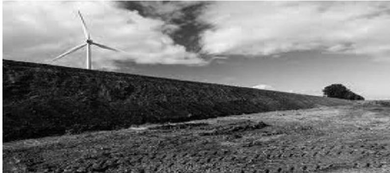
Figure 5 : Prevent intrusion of tidal water in cultivated land nearby sea shore and conserve the rain water by bunding
