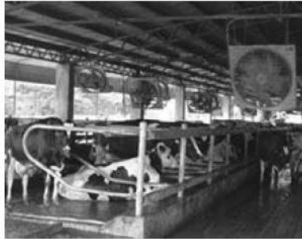
A typical Fans and spray arrangement
