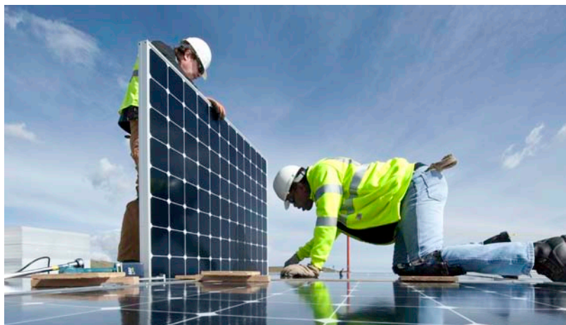
Photo by Dennis Schroeder, NREL/PIX 21499
