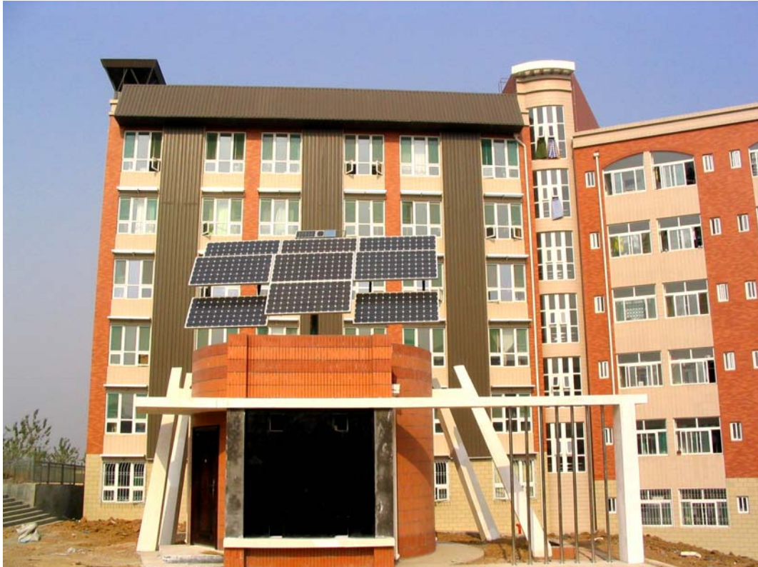
Fig.1 Appearance of the building
