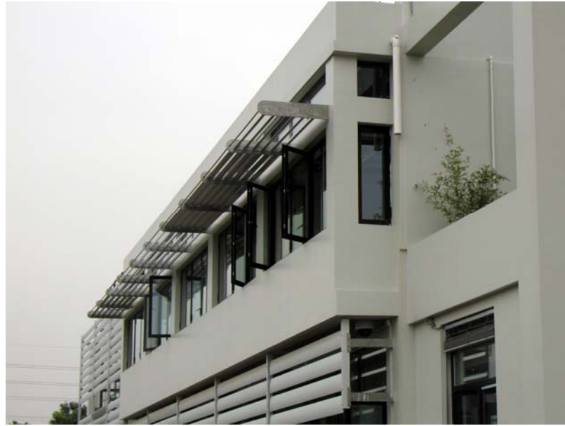
Fig.2 Adjustable horizontal sun shading devices with aluminum alloy window blind in south facade
