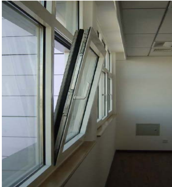
Fig.2 Thermal break aluminum frame with high performance low-E glass
