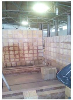
Historically, all the furnaces were lined by pressed, standard sized bricks in all the cases. So the wall thickness in all the furnaces was either 12-18 or 24 inches thick or even more, irrespective of its requirement. Anything less than 9" long was not available and hence they will use only this. Insulating materials like the Ceramic Fibre, the ULTRALITE, the Vermiculite got discovered in the last ten to twenty years.
