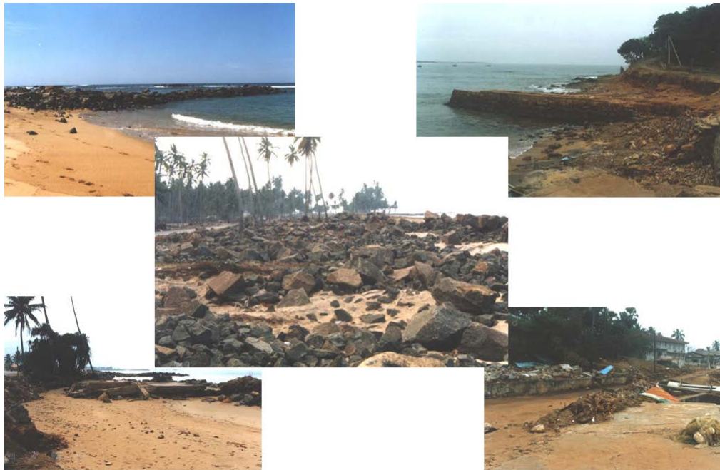
Plate 1: Disturbed revetments & groins in the Southern Coastal belt of Sri Lanka during tsunami (2004)
