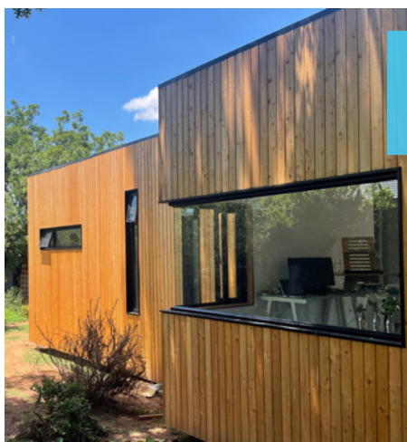
Ecomodular home modular design houses that minimise waste production in South Africa.
