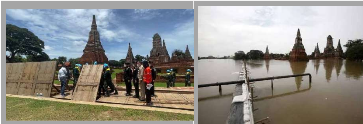
Movable flood gates being erected during pre-flood conditions and during flood situation.
