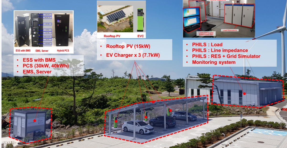
EV Charging station with RES + BESS (Jeju, Korea Institute of Energy Research)
