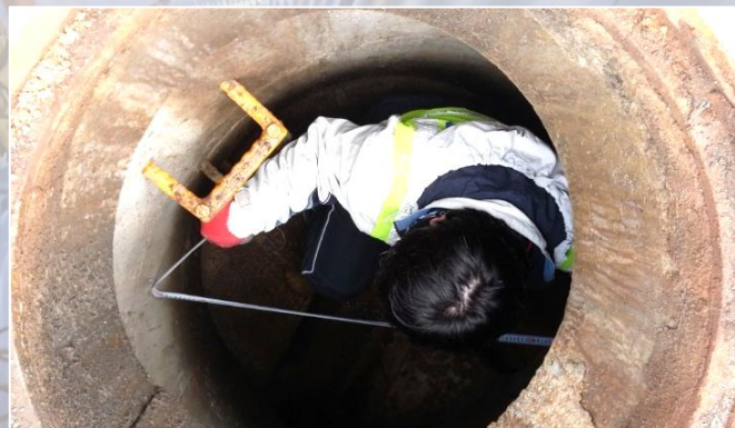
Pipe (manhole) inspection site
