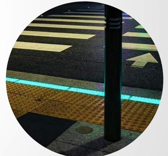
Crosswalk floor Traffic Light (Night)
