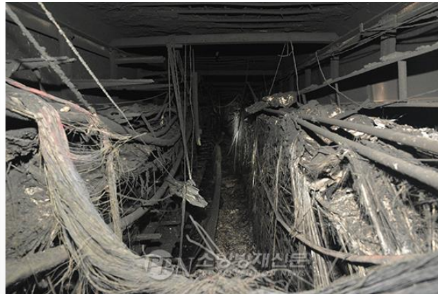
<KT Ahyeon Branch Underground Cable Fire (2018)>
