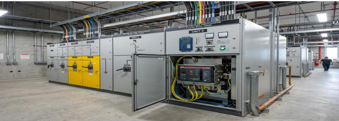
FIGURE: Modern MV Substation Switchgear & Vacuum Circuit Breaker Unit
