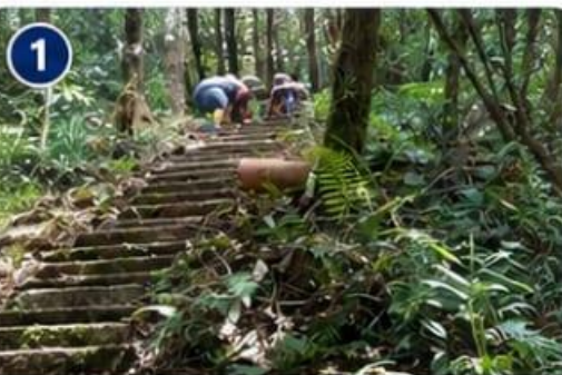
1 Site Survey & Access Preparation Tekno Park Area, Sentul
