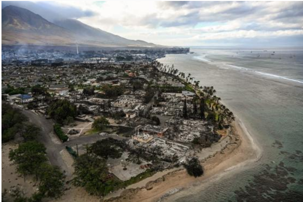
Destroyed homes and buildings on the waterfront in Lahaina, Hawaii, on Aug. 10 after wildfires tore through western Maui. Photo: Patrick T. Fallon / AFP - Getty Images
