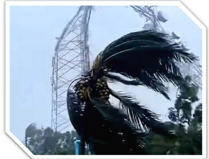
Telecom towers collapsing from cyclone in Myanmar and Bangladesh, 2023
