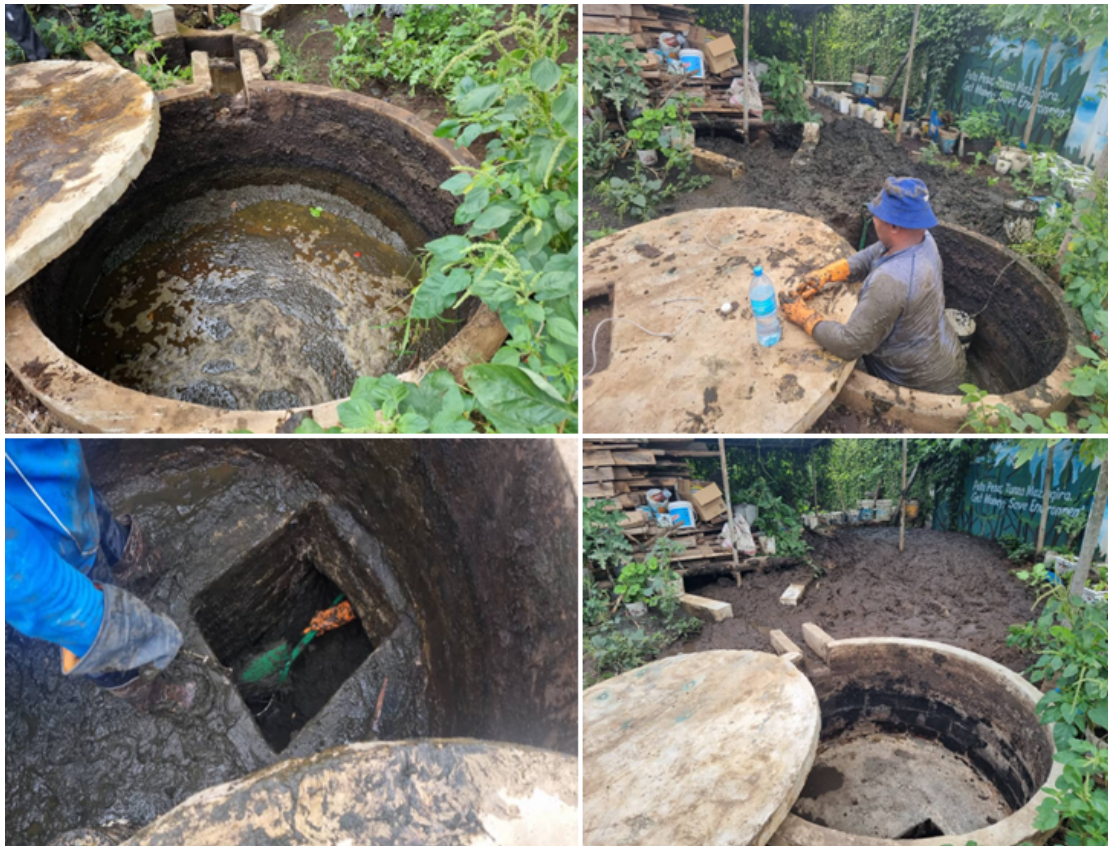
Image 2. Retrofitting work for digester tank and biogas plant, Arusha, Tanzania.
