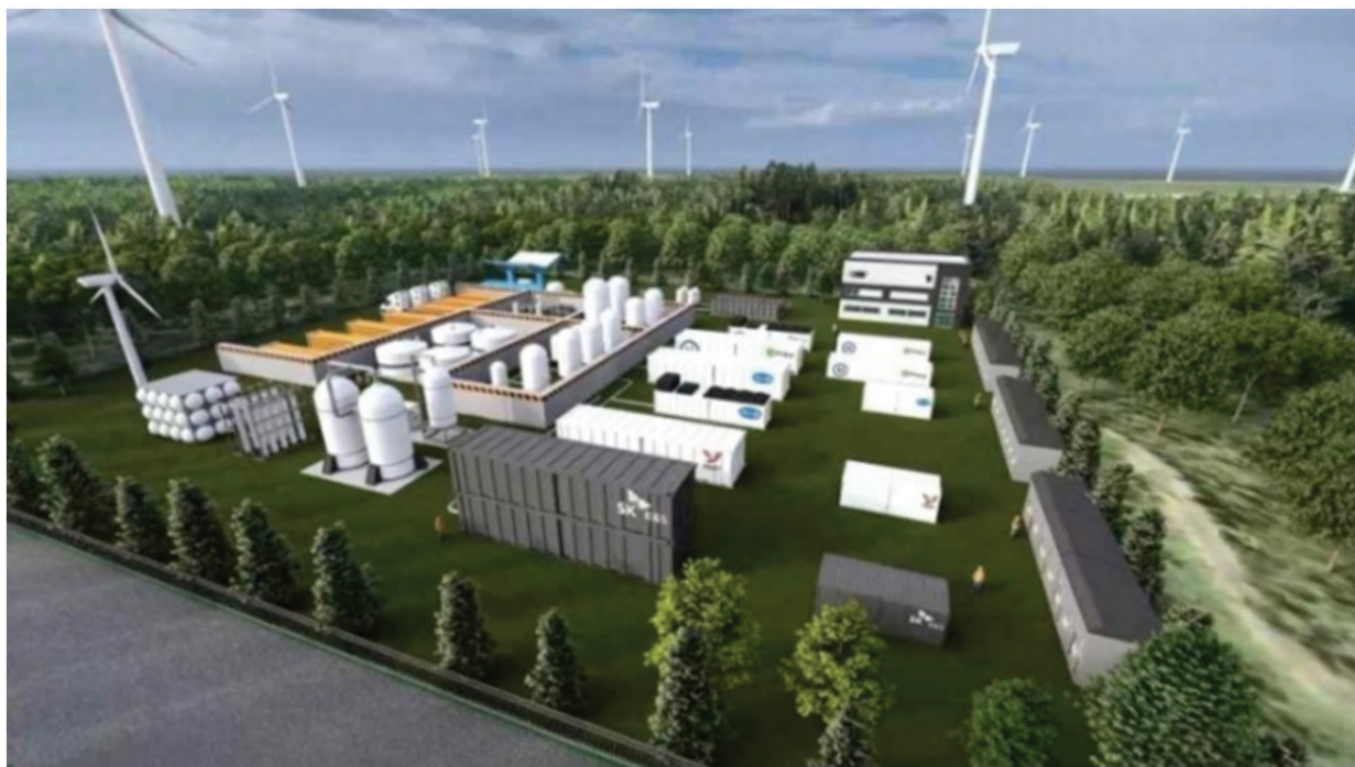
Figure 5 12.5MW Jeju green hydrogen production facility demonstration project (Ministry of Trade, Industry and Energy, 2022)
