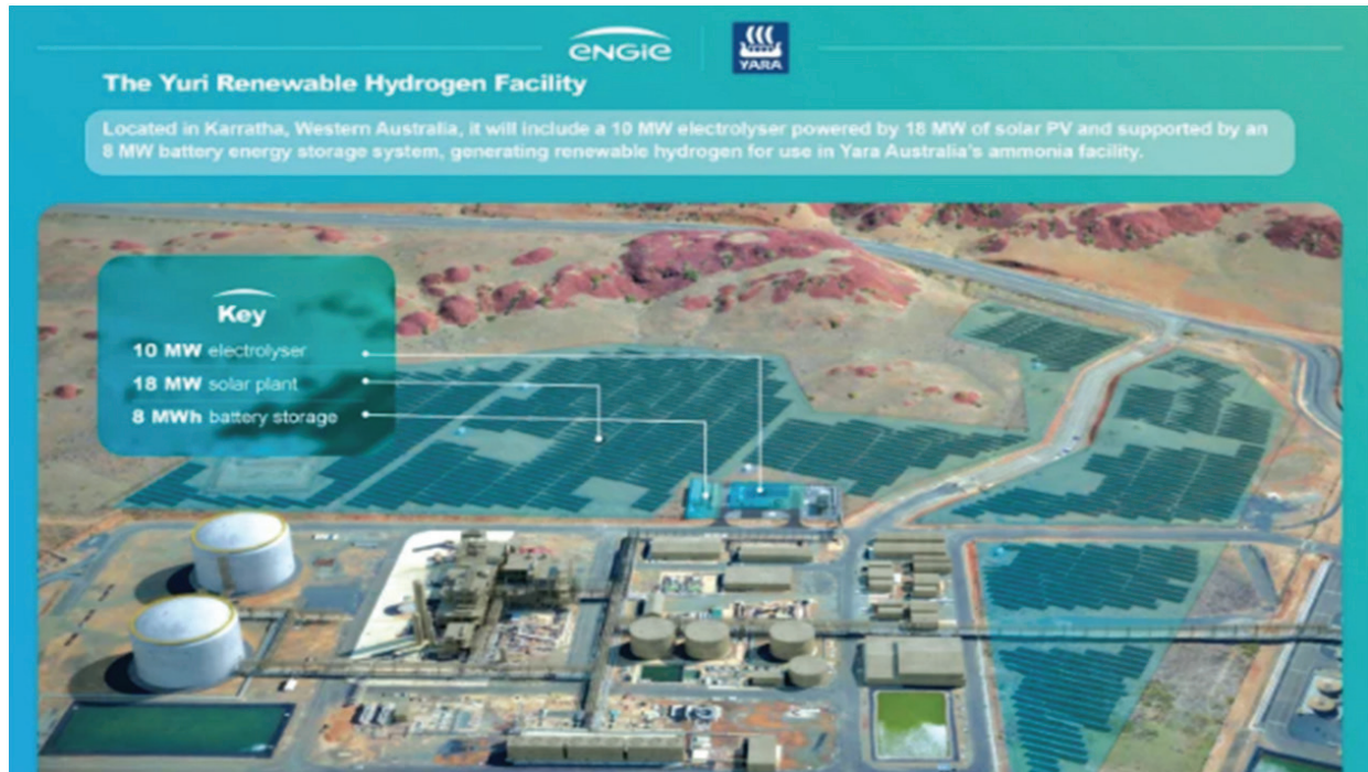
Figure 3 The Yuri Renewable Hydrogen Facility (2023)
