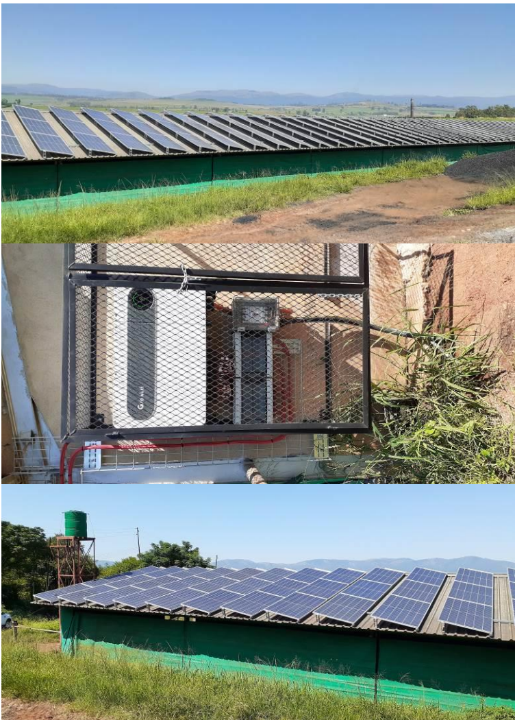
Figure 7: Example of a local solar array installed on a chicken house for cane irrigation (Hully Farm)
