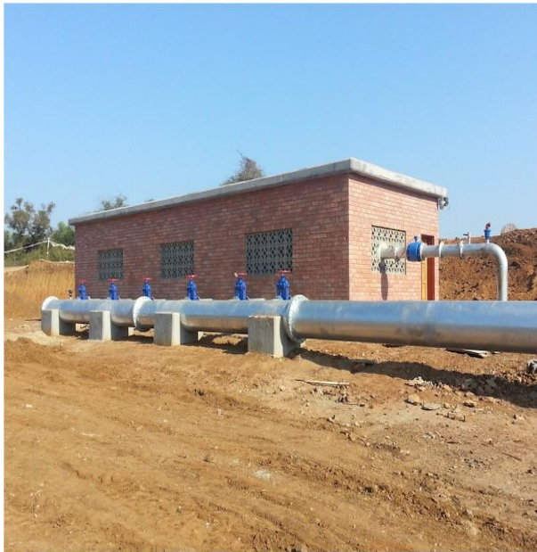
Figure 5: Discharge pipe to irrigation system
