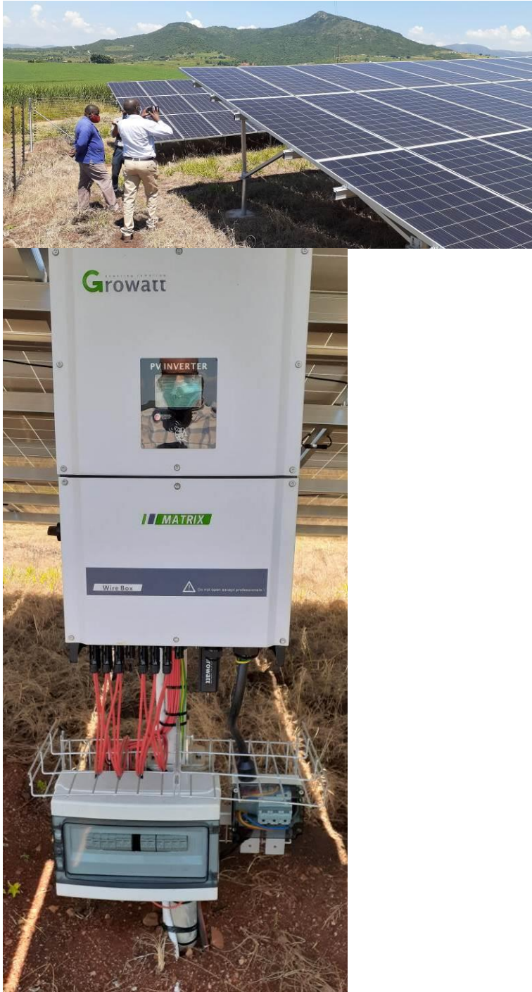
Figure 9: Example of a local ground based solar array for cane irrigation (Makamba Dad Farm)
