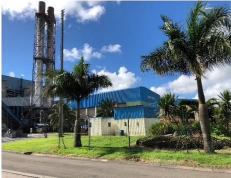
Steam Boiler and Turbine Building
