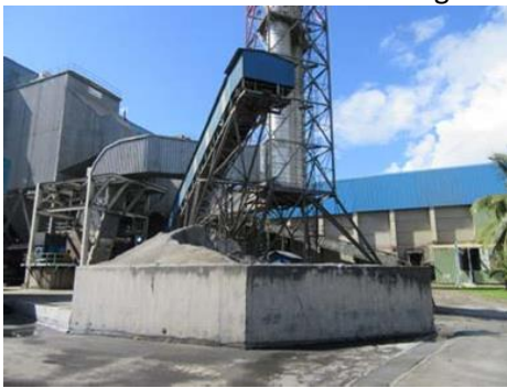
Electrostatic Precipitator, Ash Collection System
