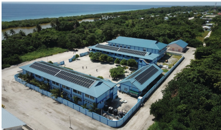
Figure 6. POSED Project (Solar PV at a School)
