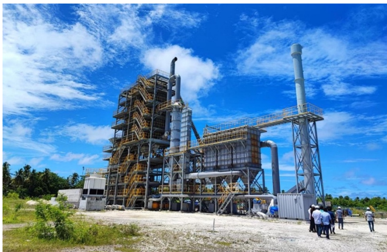
Figure 9. Addu City 1.5 MW Waste-to-Energy Plant Under Construction 17
