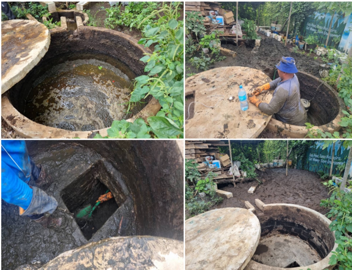
Fig. 10. The retrofitting of the biogas plant initiated with cleaning of digester tank.
