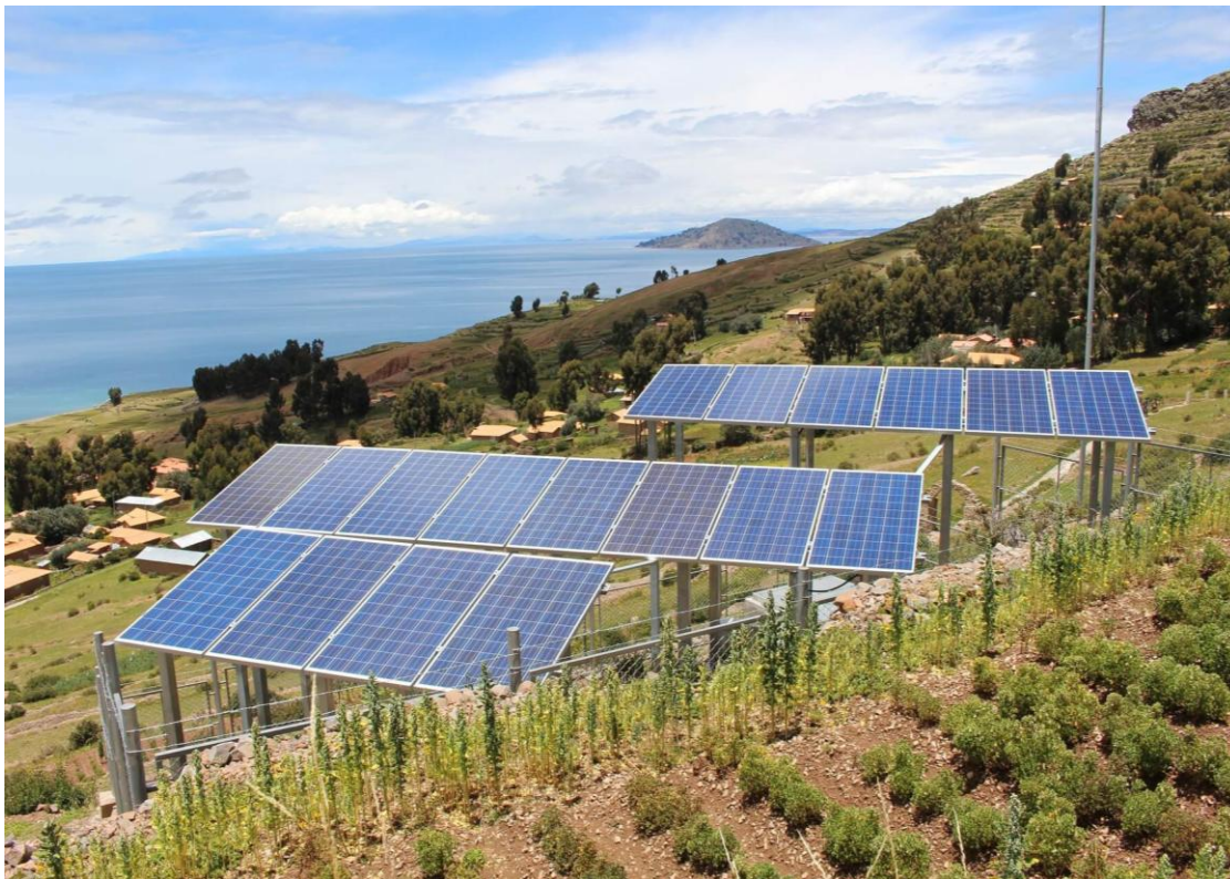
Figure 2 Example of Tilt in a Location near the Equator
