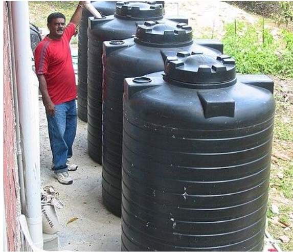
Rooftop Harvesting: Collecting rainwater from rooftops into storage tanks
