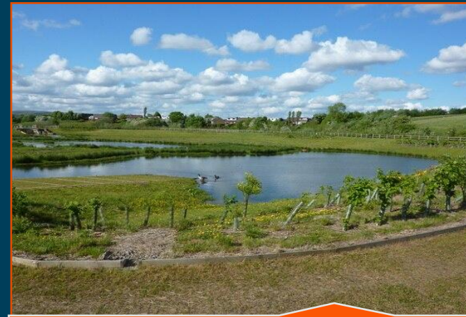
Surface ponds: Constructed ponds that capture runoff and provide a water source for crops.
