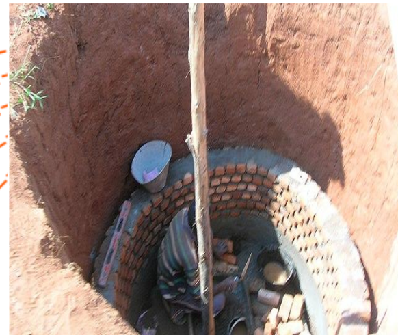
Percolation Pits: Digging pits to allow rainwater to infiltrate and recharge groundwater
