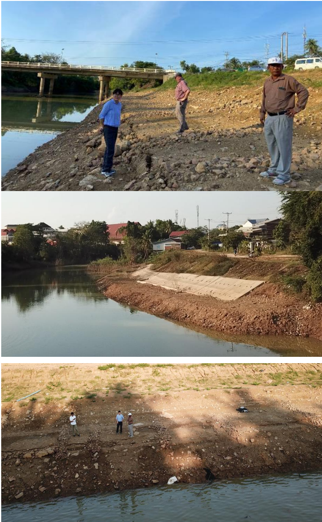
Figure 9: Site visit to a river erosion site along the Stung Sangke River
