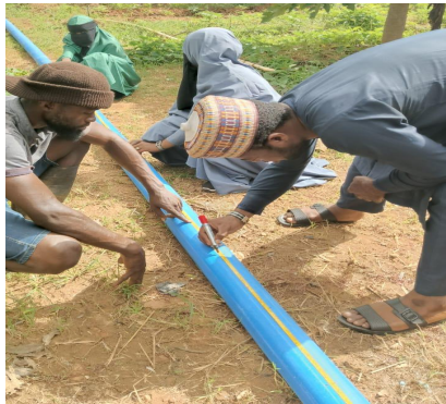
Plate 6: Showing PVC pipe used for channels
