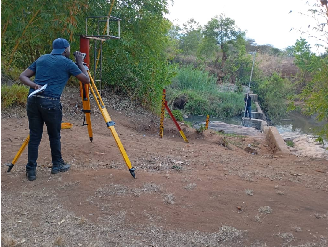
Figure 3: A technical team from the Department of Water Resources, with the support of the TA team from Water in Sight Ltd, installed and calibrated water-level measurement equipment at the Domasi River monitoring station as part of the project's equipment rehabilitation work (October 2024). DWR, TA staff and the Gauge Reader worked together to improve the reliability of the manual gauges, forming the physical backbone for digital data collection.
