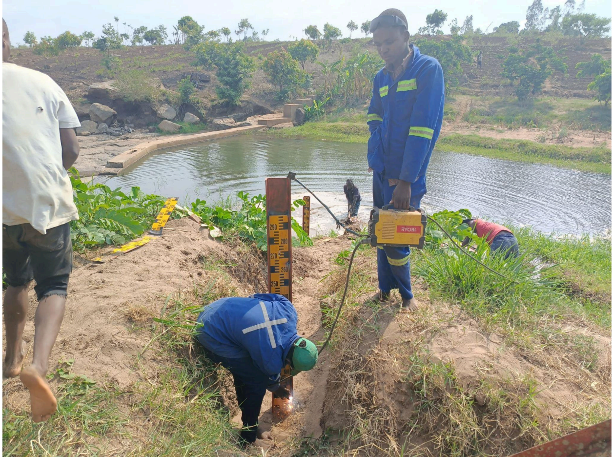
Plate is fixed and welded to the angle iron.
