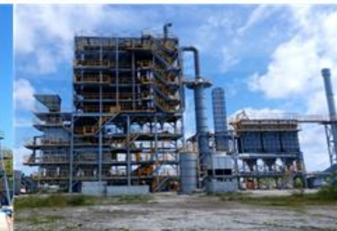
Completion of mechanical facilities
