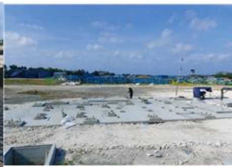
Anchor bolt installation
