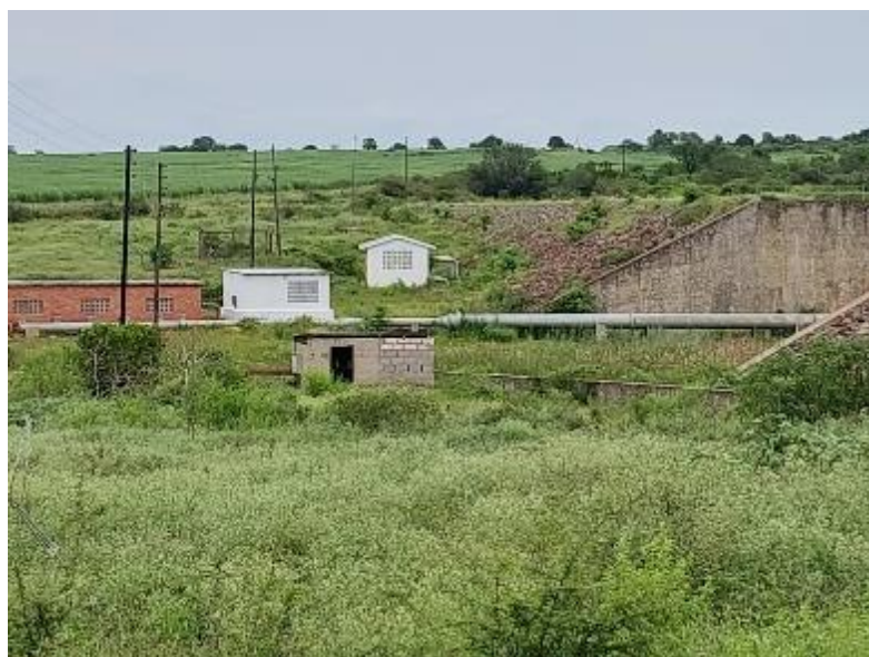
Figure 12 - Asibebahle Mbabala Pumping station.
