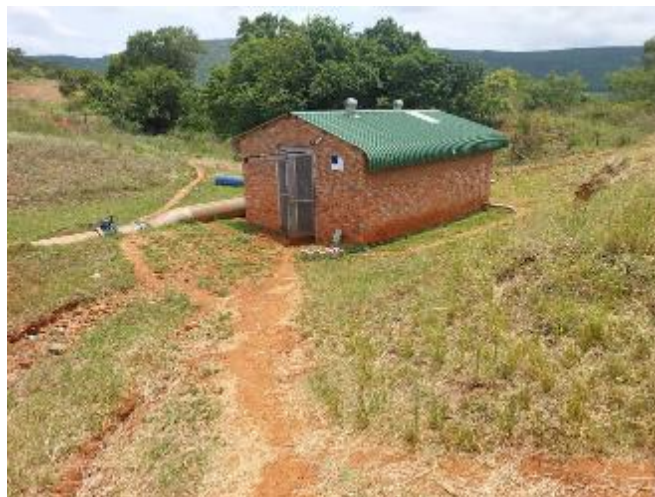
Figure 9 - Mnyangombili farm Pump Station
