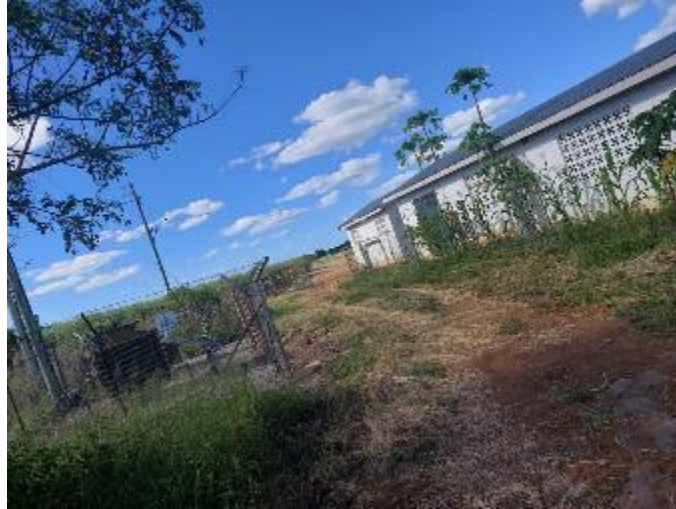
Figure 17 - Lomdashu Farm Pump Station
