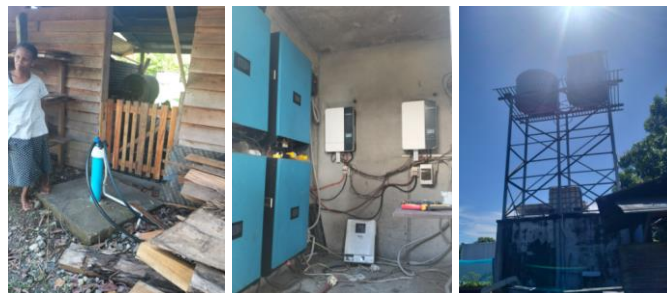
Figure 9: YWAMS, Solar submersible pump system, Burnscreek, Honiara
