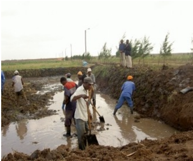
Figure 6. Construction of fish tank for aquaculture in Sofala, Mozambique.
