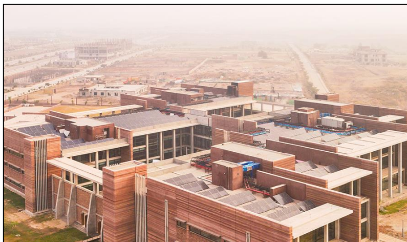
Figure 36 - PV Solar Panels, Telenor 345 Head Office
