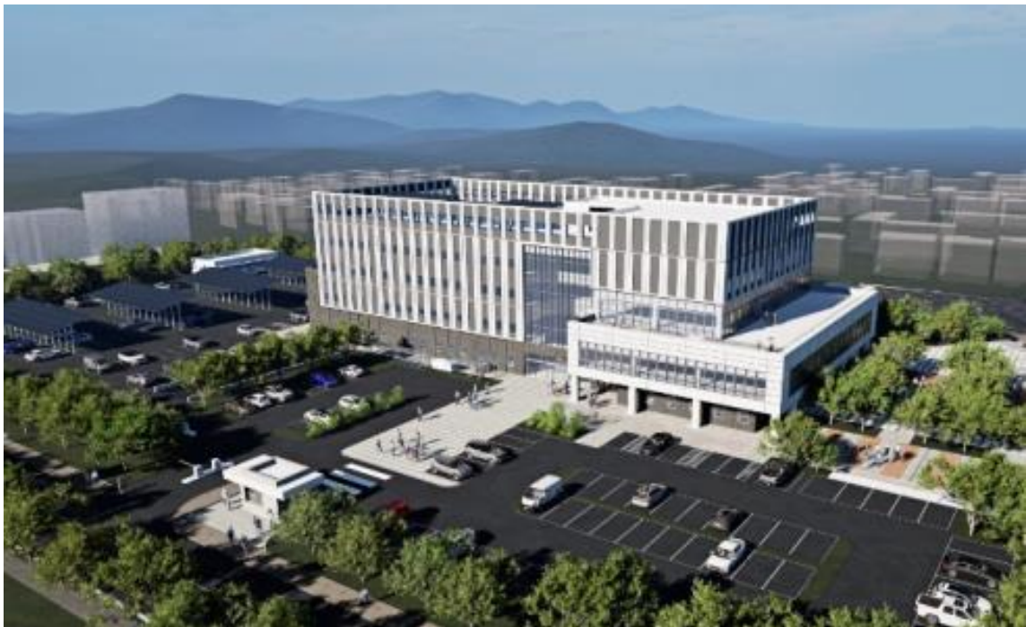
[Figure] Incheon Geomdan Police Station (Green Level 2)
