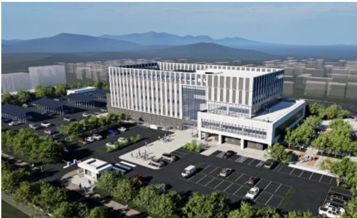
[Figure] Incheon Geomdan Police Station (Green Level 2)
