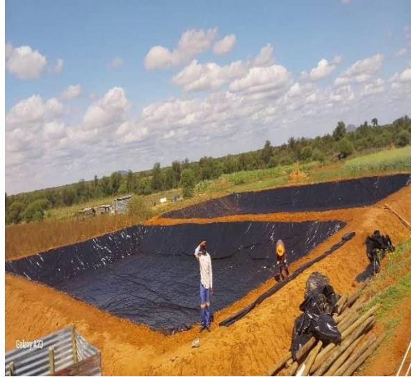
Figure 2. Earth pond farm under construction, the plastic cover, reduces infiltration.
