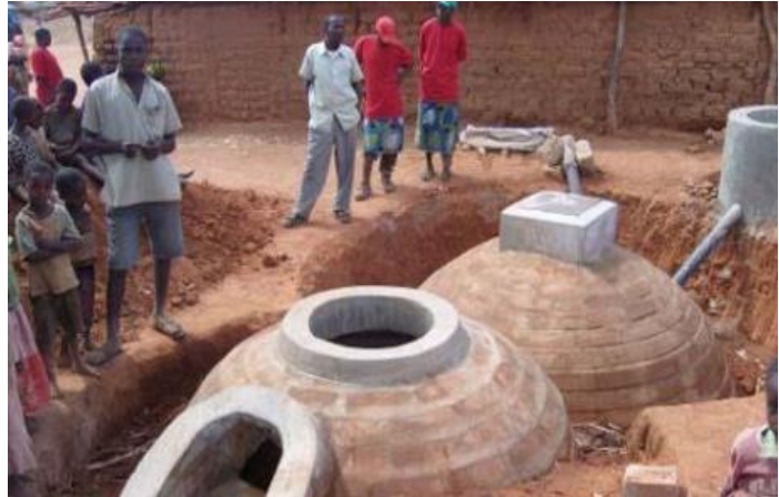
Figure 8. Fixed-roof biogas installation (greenempowerment, 2023).
