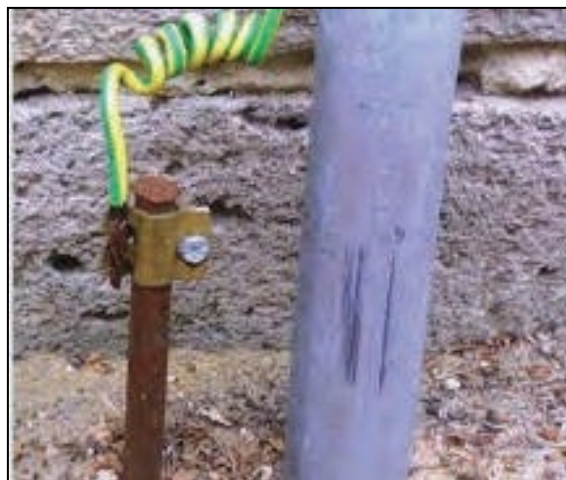
Figure 7: Earthing/Grounding for Lightning Protection
