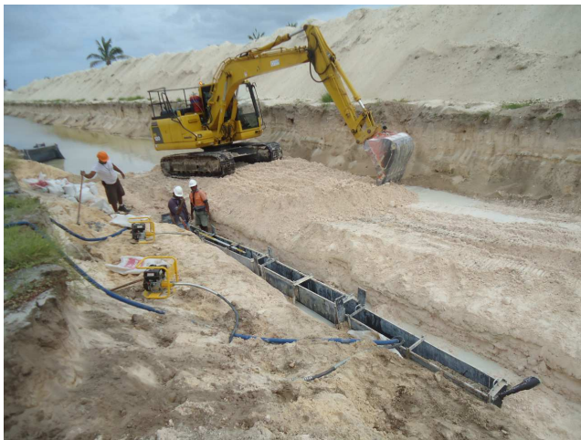
Installing the gallery
