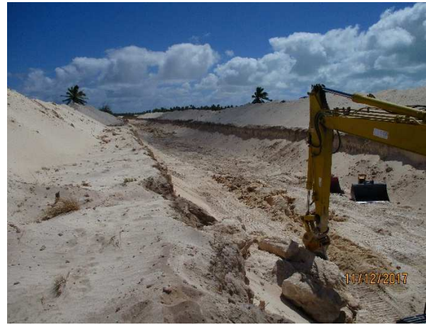
Excavating for the pipe
