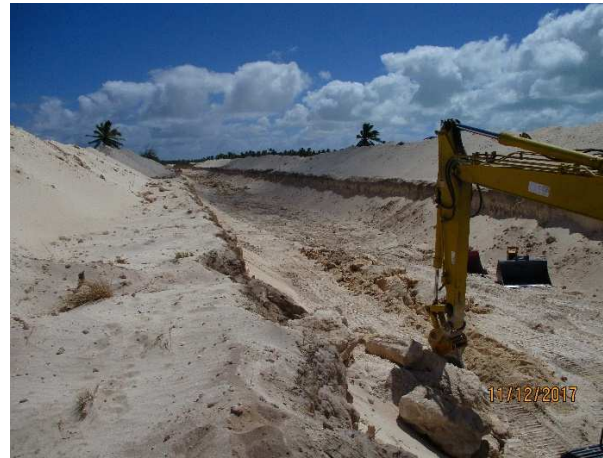
Excavating for the pipe
