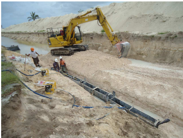
Installing the gallery
